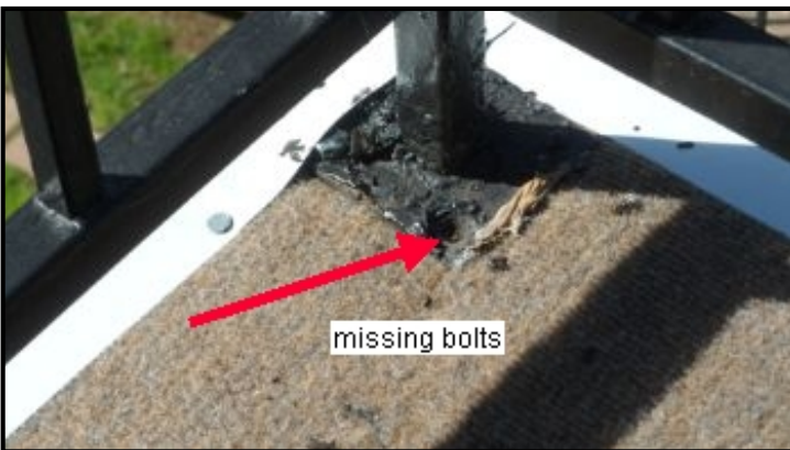
Missing bolts at Multiple locations
